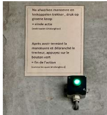
Figure 4 - Green button next to the quay gate. Driver presses this button after arriving at quay.
