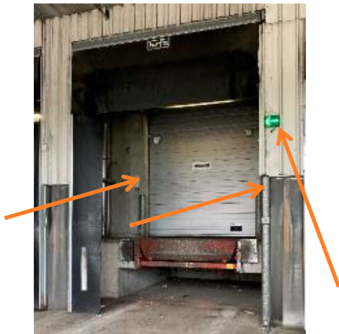
Figure 3 - Quay with the illuminated green arrow. The green button is located along one of the two sides of the gate.
